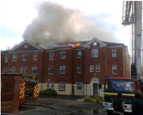
Electrical installations in poor condition present risks of fire as well as electric shock.
