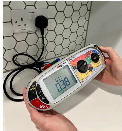
Electrical tests being carried out.
