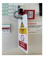
The practice of placing insulating tape over a circuit-breaker to prevent inadvertent switch-on is not an acceptable means of securing the device in the OFF position. Such unsafe practice will not achieve compliance with the Electricity at Work Regulations 1989.
