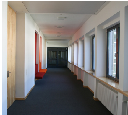
Typical communal corridor containing lighting and power.
