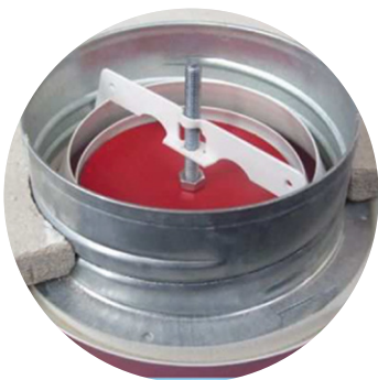
Fire rated Ceiling Air Valve installed before a fire
