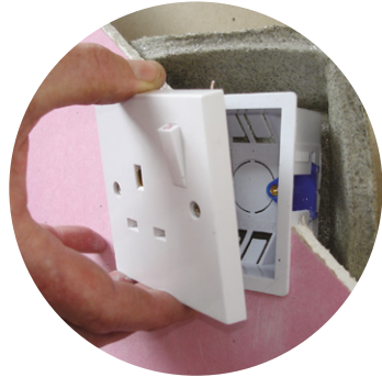
Fire and acoustic rated covers fitted behind dry lining box (Photo courtesy of Tenmat Ltd)
