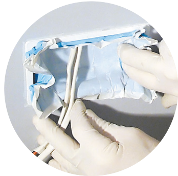
Intumescent pad being installed in a dry lining box (Photo courtesy of Knauf Drywall)
