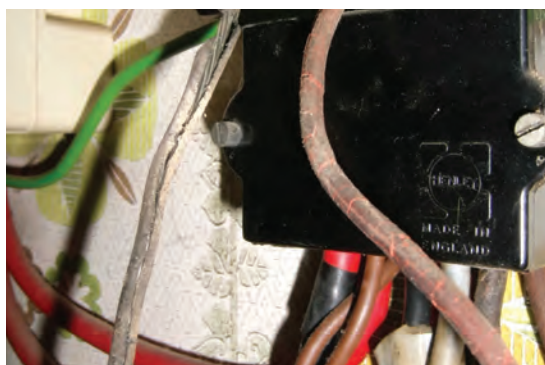
Live parts exposed to touch
