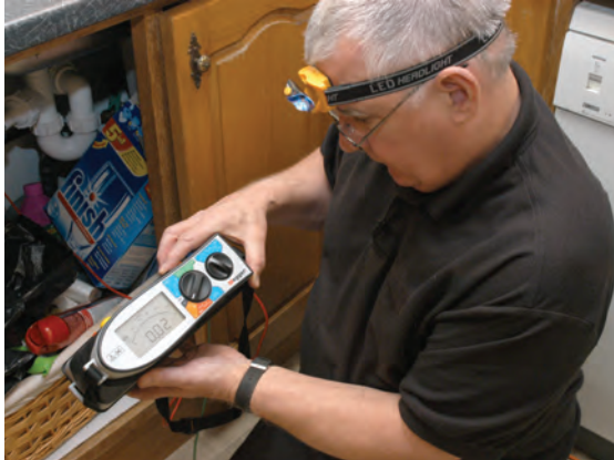
A continuity test being carried out
