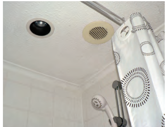
Recessed luminaire above a bath (outside the zones)
