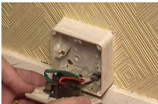
Inspecting a socket-outlet
